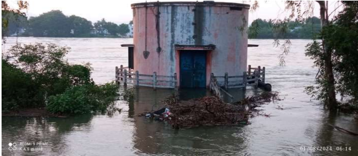
CWSS to Kadappanallur- water level reached floor level of the pumproom
