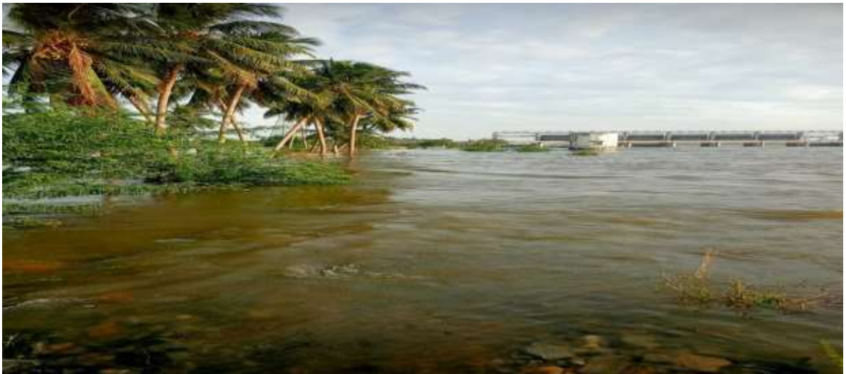
CWSS to Muthamapalayam – EB supply affected and Pumproom is in inaccessible condition
