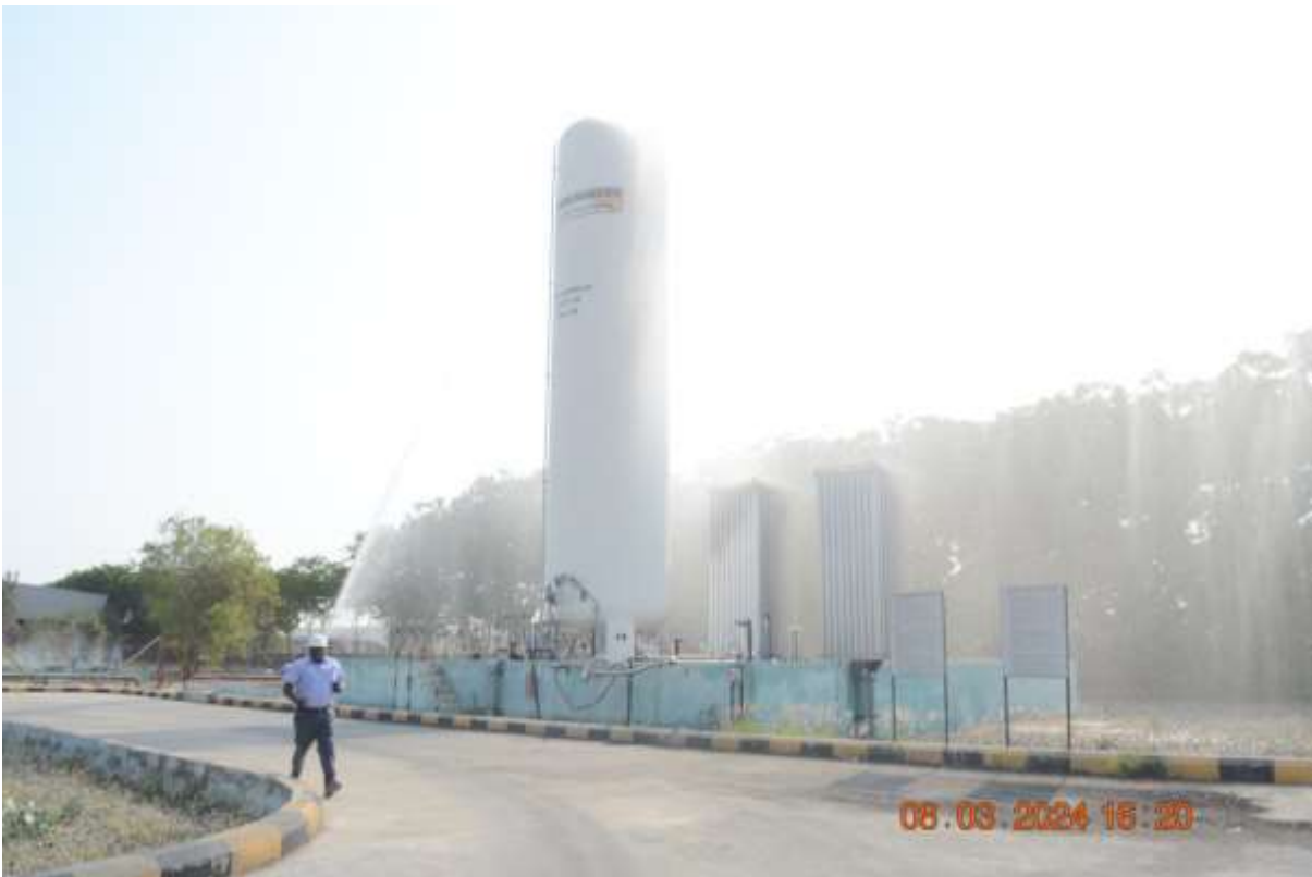
After siren raised all the employees evacuating from the factory to Safe Assemble Point #2
