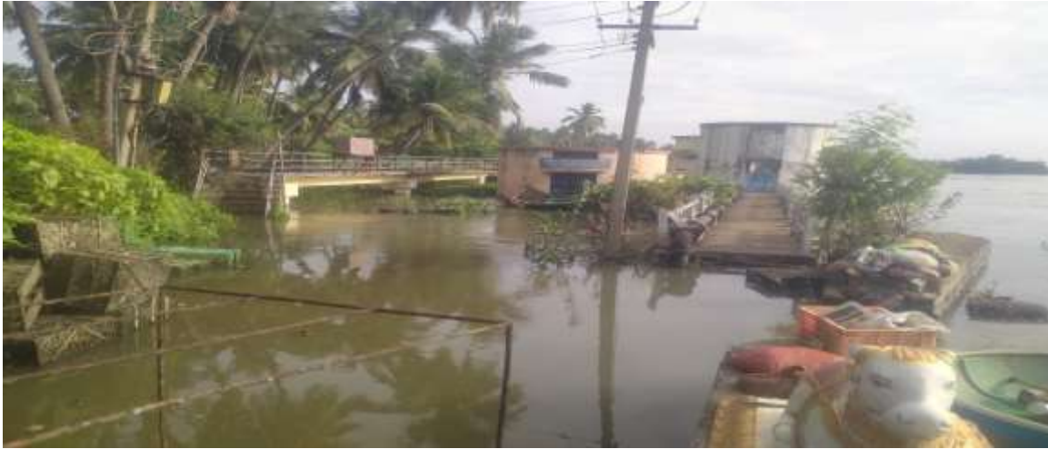
CWSS to Chennimalai-Collection well (Old) submerged in headworks at Konavaikal
